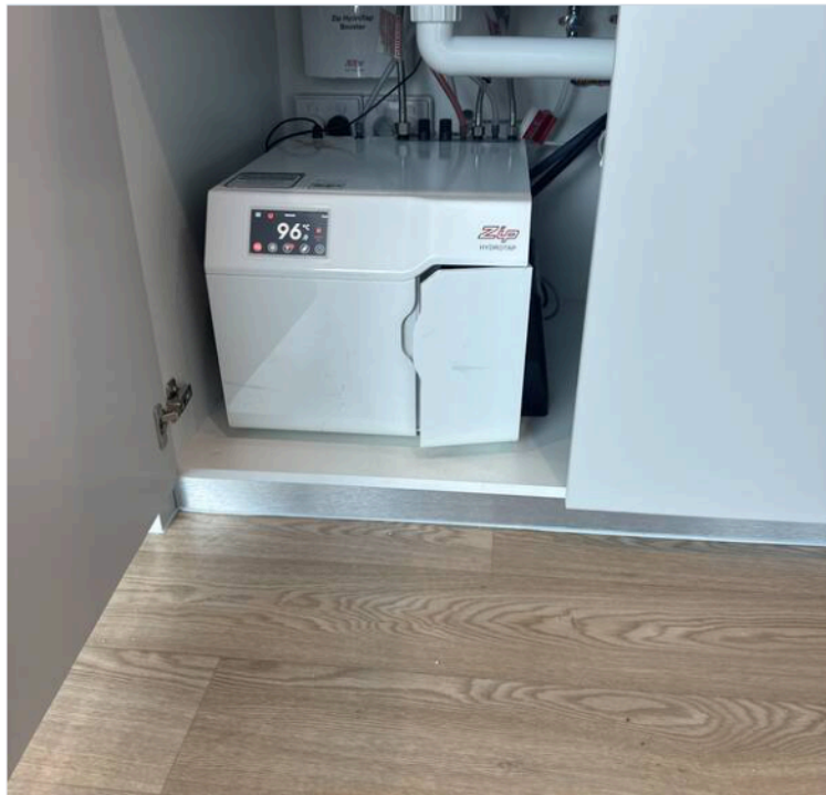
Ref 13a · #13 Vent for zip tap to be installed for: Plumber
