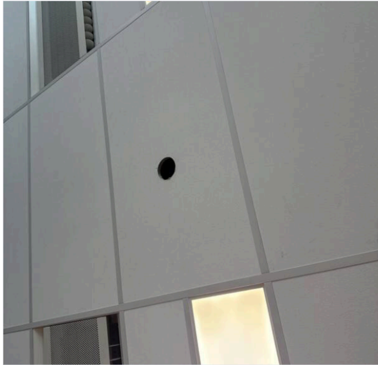
Ref 17a · #17 Replace tile for: Carpenters
