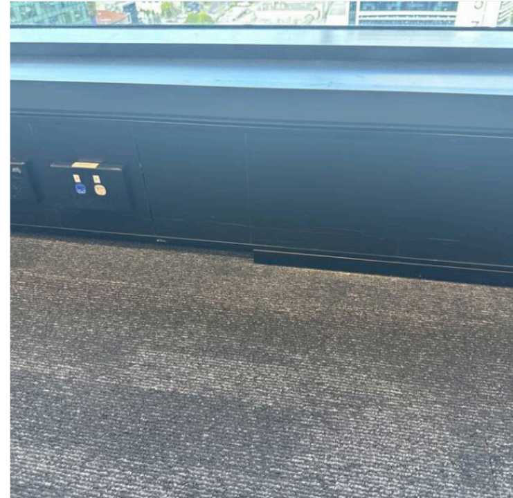
Ref 3a · #3 Black filler under truncated skirting not fixed in place for: Carpenters
